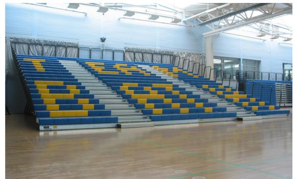
Although the floor will compress when pulled out under the weight of the seating units it will return to its normal position once the load is removed. In some cases we may strengthen the area under the wheel runs if the bleacher seating units are particularly heavy.
