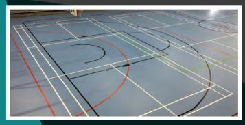
DYNAMIK A4 AREA ELASTIC SPRUNG FLOOR FINISHED IN SEAMLESS
