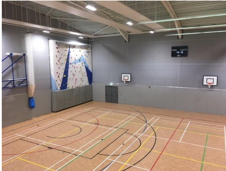
DYNAMIK A4 area elastic sprung floor finished in Sports Vinyl as installed at Badminton School.
